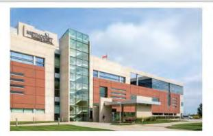
Expanded wing: Methodist Women's Hospital was built with expansion in mind. Footings in the roof surfaces allows for outward and upward growth. The NICU expansion extends off the existing third floor space which faces southeast toward Dodge.
